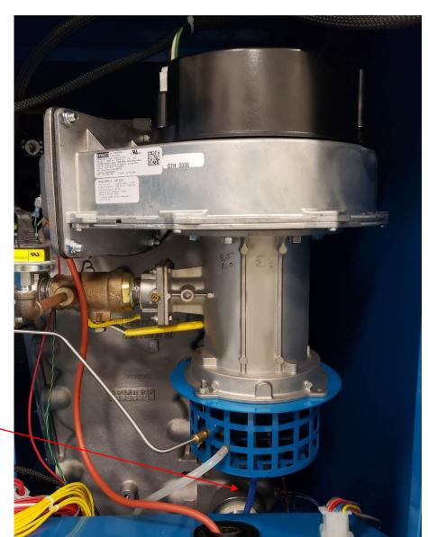
Unit must be leveled from the bottom of the intake basket.
